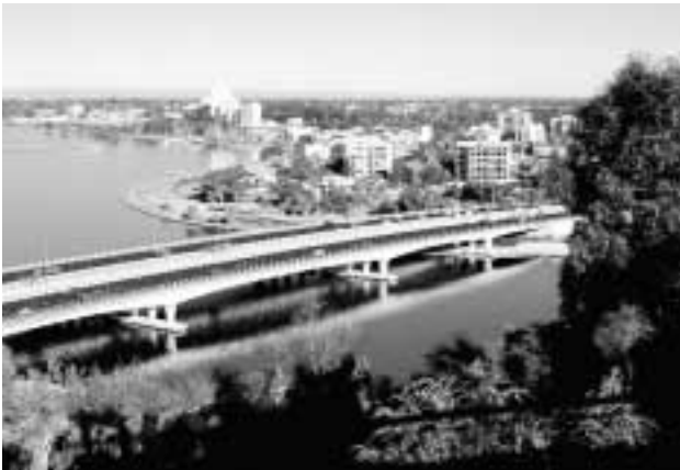
The Narrows Bridge, spanning the Swan River. Photo: John Chapman/AAP Image
